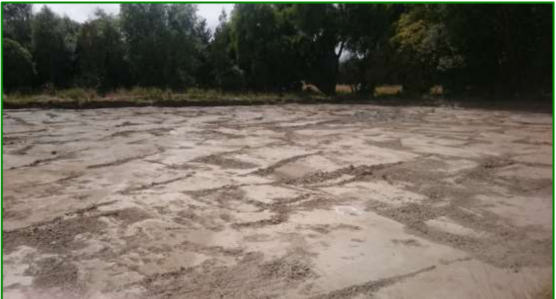
A 3-4m grid of XRF tests showed arsenic well below the SGV across the rest of the excavation.
