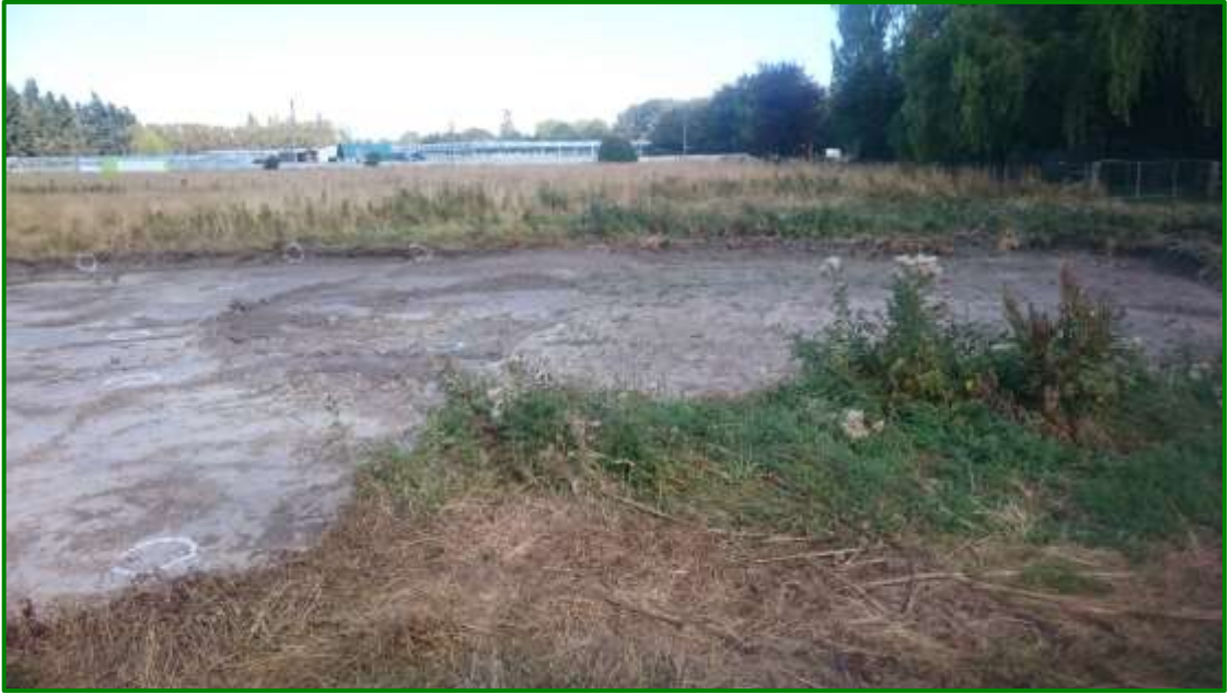
Final extent of excavation in burn pile area, 'O' marks XRF readings below SGV
