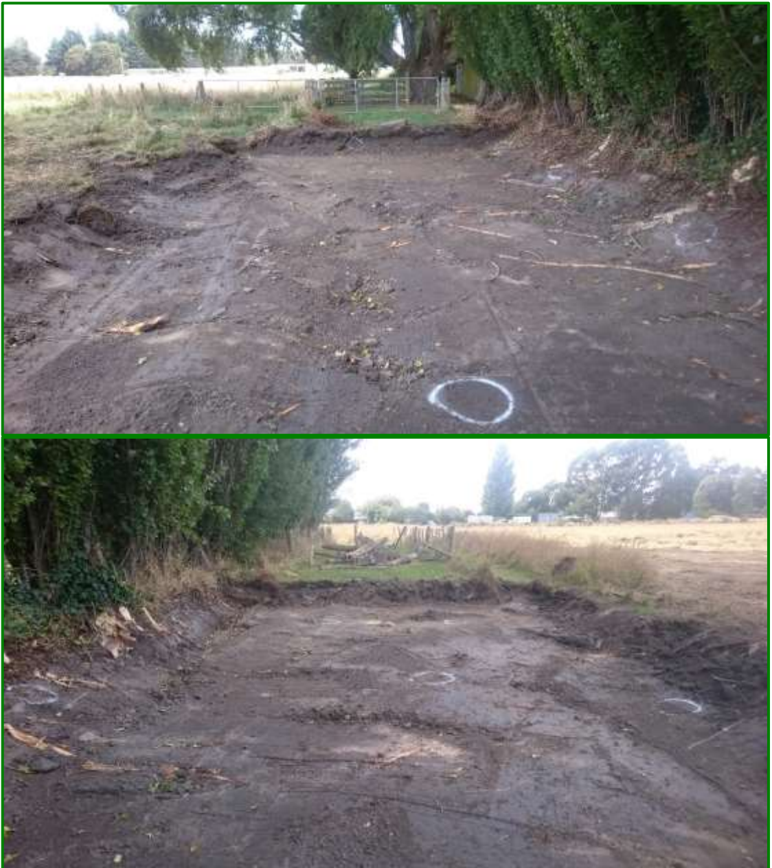
Excavated sheep drafting yard area, 'O' marks XRF test locations with arsenic below SGV
