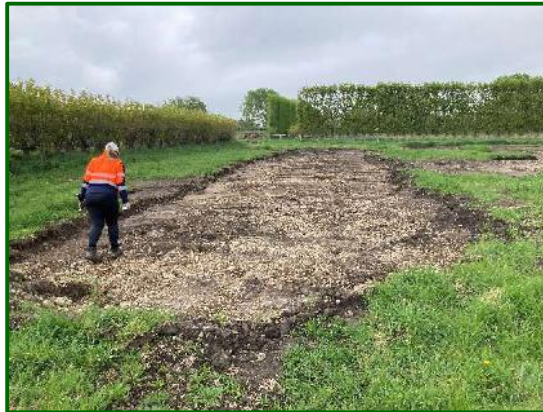
Photo 7 – XRF testing after stockpile removed from site
