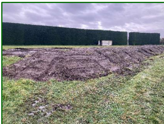
Photo 5 – Stockpiled excavated soils
