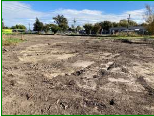
Photos 6-7: Final excavation of ACM impacted soils
