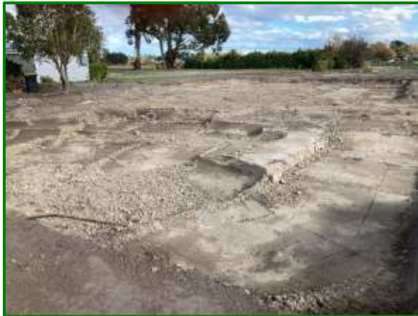
Photos 12-13: Eastern area of heavy metal contamination with XRF test locations, some excavation still required on eastern wall
