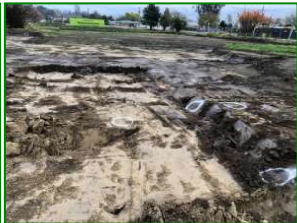
Photos 14-15: Final excavation of eastern area of heavy metal contamination (eastern wall and around VS_Y16)
