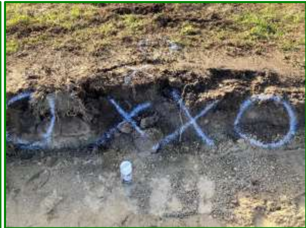
Photos 12-13: Eastern area of heavy metal contamination with XRF test locations, some excavation still required on eastern wall
