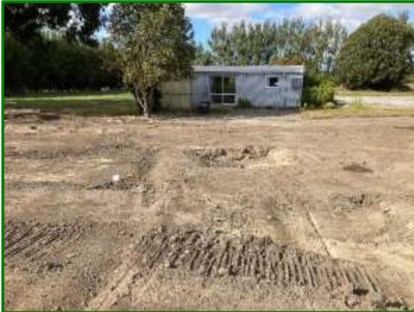
Photos 4-5: Parts of excavated area of ACM impacted soils on 4 Glovers Road including deeper pits
