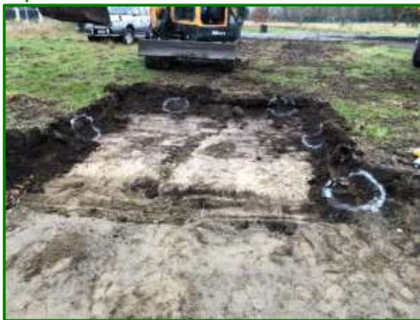
Photos 14-15: Final excavation of eastern area of heavy metal contamination (eastern wall and around VS_Y16)
