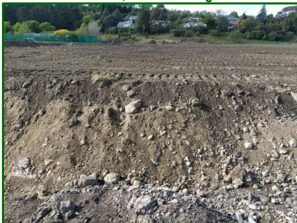
Photo 3 – 15/10/2020; topsoil and sub-base layer
