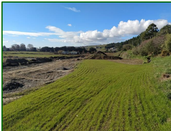
Photo 2 – 13/07/2021; Lot 62 looking east
